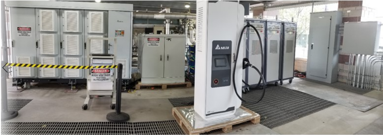
Figure II.1.11.7 400kW XFC Setup Front View (SST, Charger Power Cabinet, Dispenser, and DCE from left to right)
