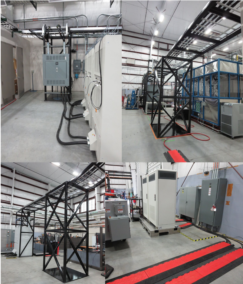
Figure II.3.3.9 Electrical connection between grid emulator and XFC in ESL
