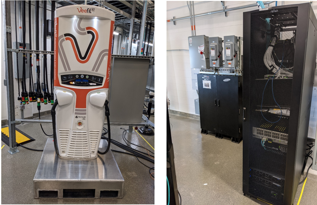
Figure II.2.2.6 Tritium fast charger (on left) and Samsung energy storage system with OPAL 5707 server rack (on right)
