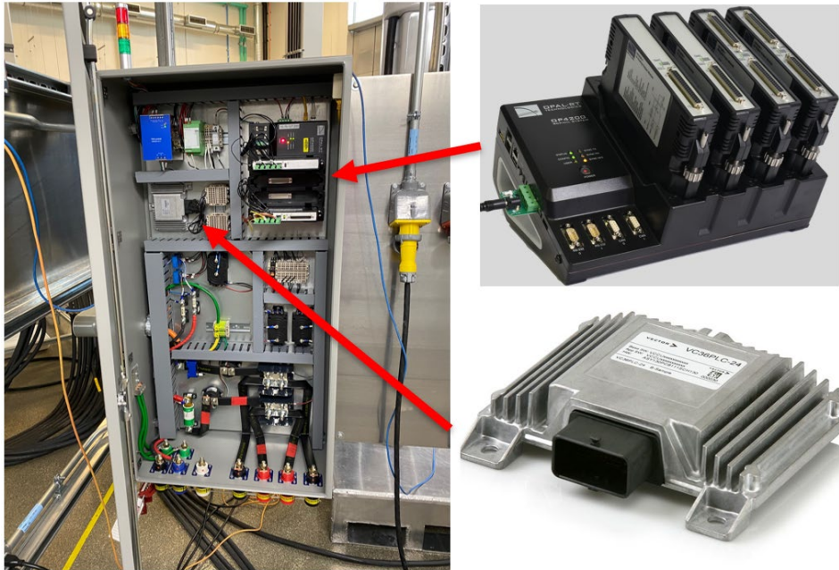
Figure II.2.2.3 Completed CCB cabinet
