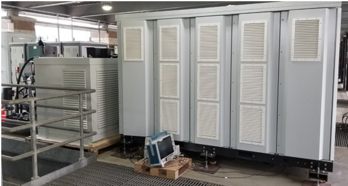
Figure II.1.11.8 400kW XFC Setup Rear View (DCE Cooling System, Buck charger, SST from Left to Right)
