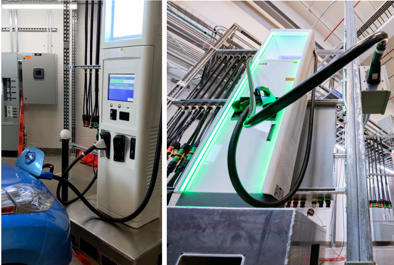
Figure II.3.6.8 BTC Power 350 kW charger connected to Nissan LEAF (left) and ABB Terra HP 350 kW charger connected to vehicle emulation hardware (right)
