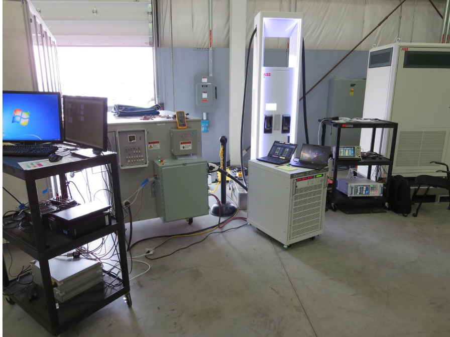
Figure II.3.3.4 ABB TerraHP (350 kW) XFC charging the CCS vehicle charging emulator in INL's EVIL
