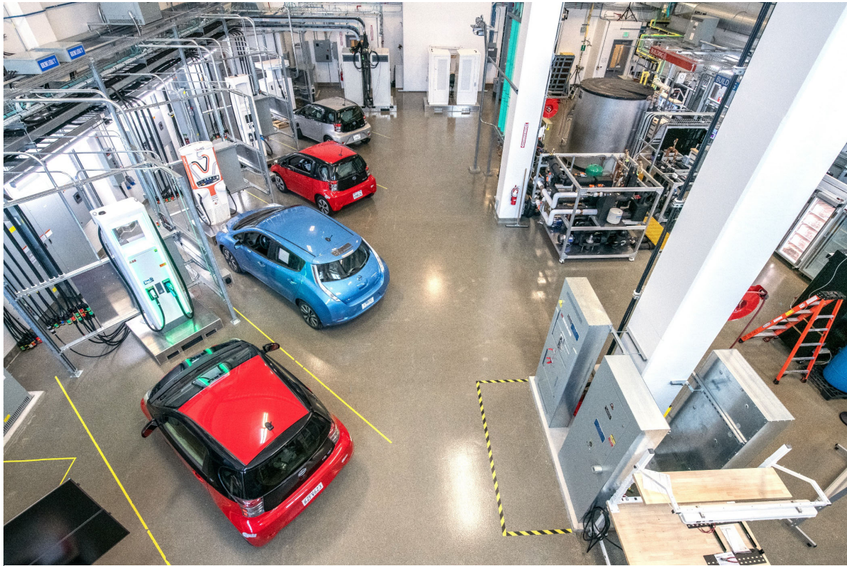
Figure II.2.2.2 Electric Vehicle Research Infrastructure (EVRI) on right with four vehicle parking bays each with both DC and AC charging and Commercial Building Research Infrastructure (CBRI) on the left with building loads and emulation
